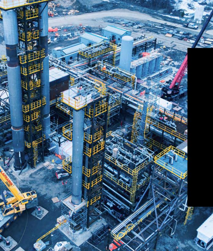
The Prince George Refinery is a light oil refinery owned by Tidewater Midstream & Infrastructure Ltd. The project requirements were connection design, detailing, fabrication and shop assembly.
